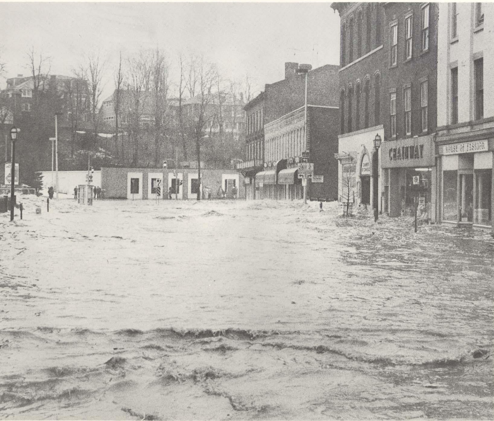
Walton Street awash with flood water.
